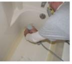
9. Vacuum all debris from sanding and wash the bottom of the tub or shower with solvent .
