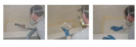
10. Put on gloves and mix together parts A and B of adhesive (1:1 ratio) into supplied container. Mix thoroughly. (Appx. 1 minute)
