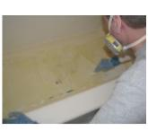
12. Holding at both ends, first place the center of the inlay down in tub, followed by the ends and adjust to the permanent location.
