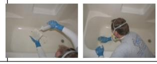
2. Position the inlay on the bottom of tub/shower and adjust to its final location.
